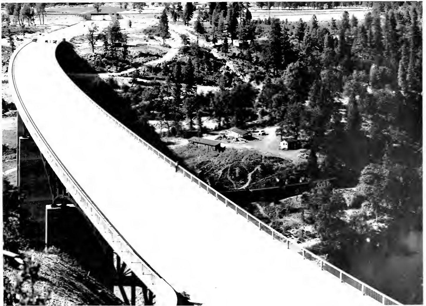
View of 50-foot roadway of Antler Bridge built on 850-foot radius curve to carry relocated 4-lane divided highway
